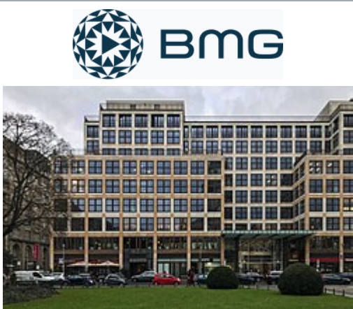
Quartier 205 in Berlin Mitte , where the headquarters of BMG are located (2018)
